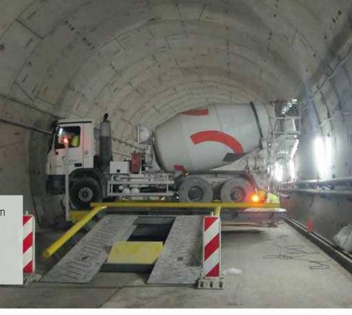
Movable revolving platform to turn trucks inside tunnels and to use at civil work. Load 50 tonnes.
