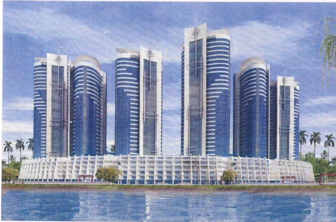
HYDRA AVENUE TOWERS AL_REEM ISLAND RT3 PLOT C4:C9
