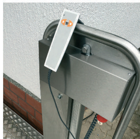
Standard operation: hand control unit on a flexible spiral cable with UP/DOWN button
