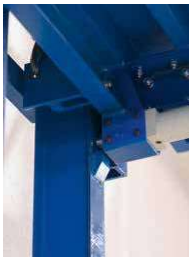
Details of the anti-creep latch
