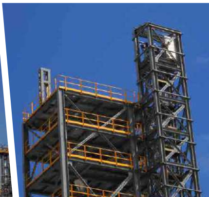
HELPE - Tessaloniki TTD ( Top Traction Drive ) ATEX - Explosion Proof T= 46m - 0,63m/s - 1.300kg
